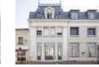
MONTEARAU THE AGENCY Accommodation
